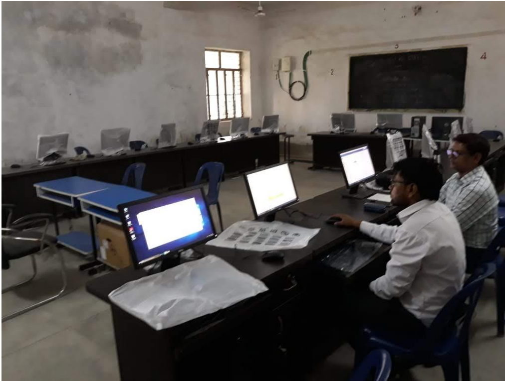
Checking the Installation
